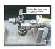
The Municipality accepts no responsibility for damages that result if the service side valve lever is not closed when the curb stop is opened in the spring.
